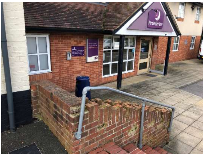
Photo 5: View of the eastern façade of the 'Premier Inn' building.
