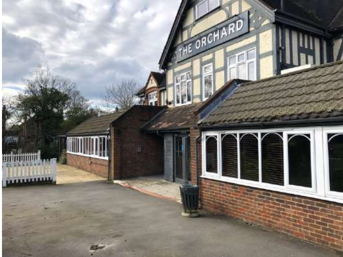
Photo 1: Southern façade of the former Beefeater 'The Orchard' building.
