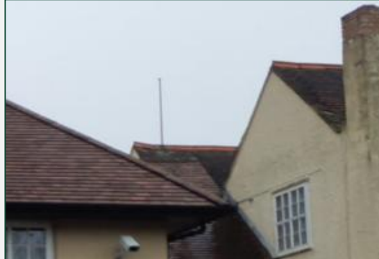
IMAGE 6: BUILDING SIDE VIEW
