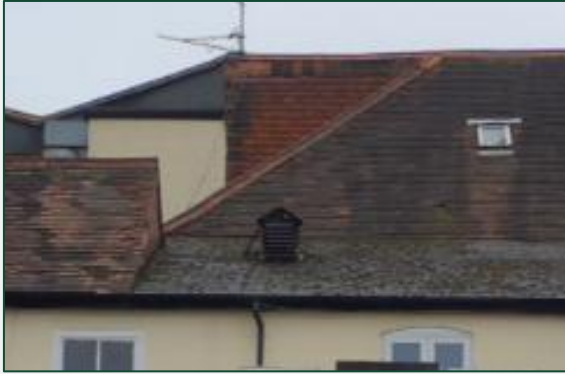
IMAGE 5: BUILDING REAR VIEW
