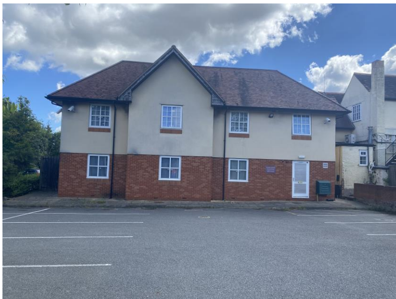
Plate 14: Looking E at the W-facing elevation of the hotel section of the Orchard.
