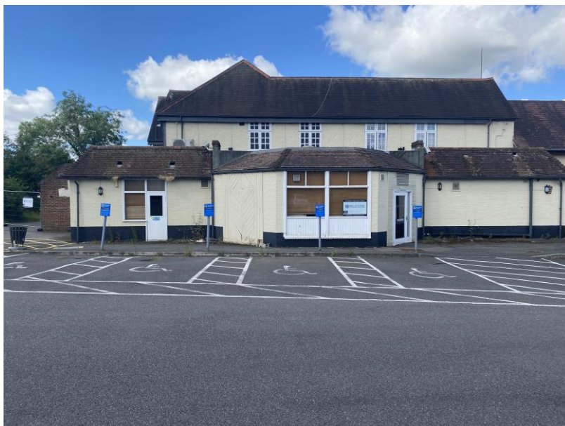
Plate 10: Looking W towards the southern part of the E-facing elevation.
