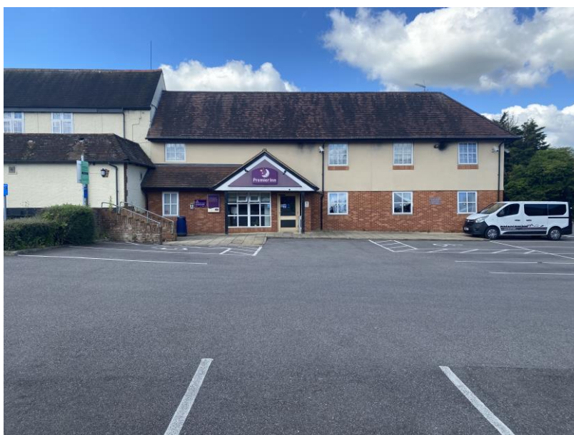
Plate 11: View W looking towards the northern part of the E-facing elevation.
