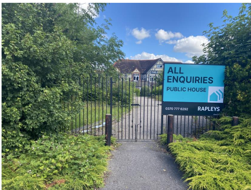
Plate 5: Looking N towards the Orchard's S-facing elevation, taken from the pedestrian access off the B466/Sharps Lane roundabout.
